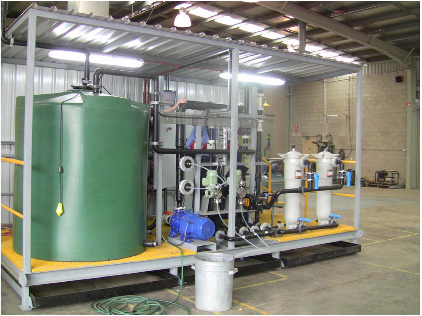
Figure 1 : Completed well house unit undergoing wet testing
